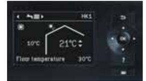
Display of the Vitotronic 200 heat pump control unit
