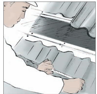
2. Measure roof & remove tiles.
