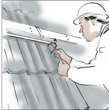
6. Fix rail to brackets. 7188482 & 7175265/7188483 & 7194423
