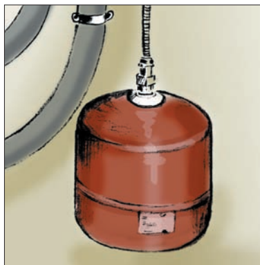
D. Check & adjust nitrogen pressure.
