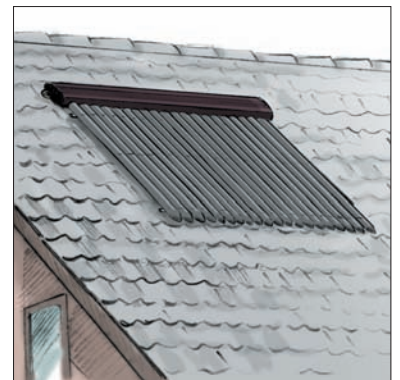
16. External installation is now complete.
