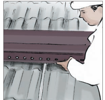
7. Fix header to rails. 7188858/7188859
